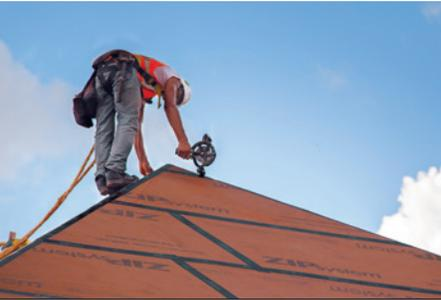
ZIP System® sheathing and tape delivers a sealed roof deck and integrated underlayment built into every panel. Build with confidence knowing your roof has a continuous water-resistive barrier, and capture the financial and scheduling benefits of immediate rough dry-in with ZIP System™ flashing tape.
