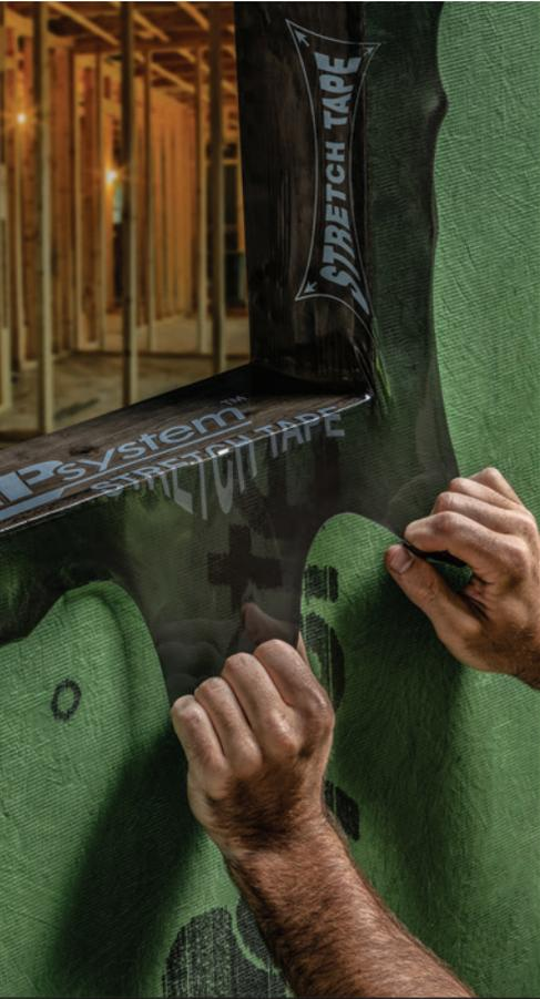
ZIP System™ stretch tape easily stretches to fit sills, curves and corners with a single piece without having to piece tape segments together. Made of a high-performance composite acrylic, the tape conforms to challenging applications and locks out moisture even over mismatched surfaces.
