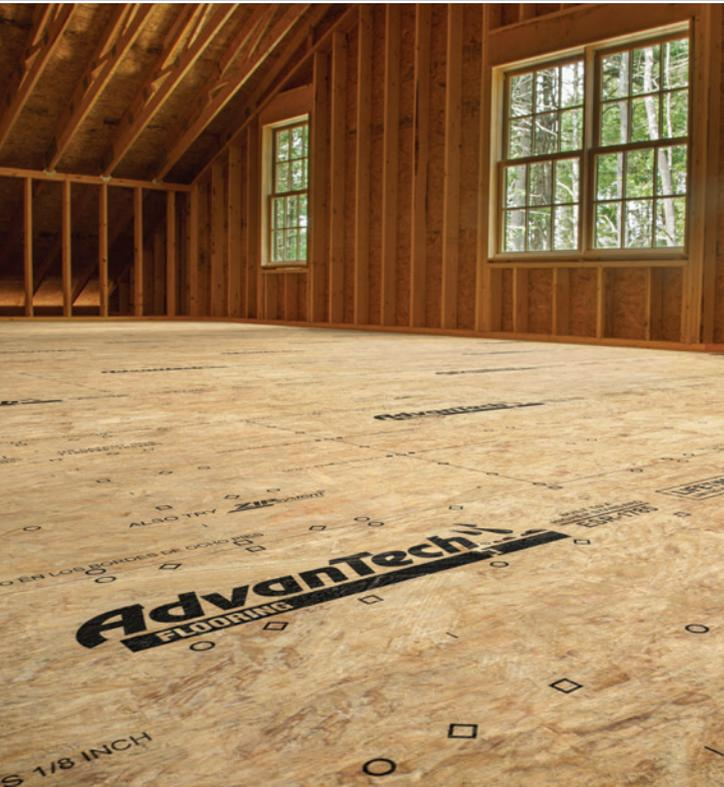
With our precision engineered tongue and groove system, AdvanTech® subflooring panels help deliver a secure fit for dependable edge-to-edge support to prevent movement that can cause squeaks.
